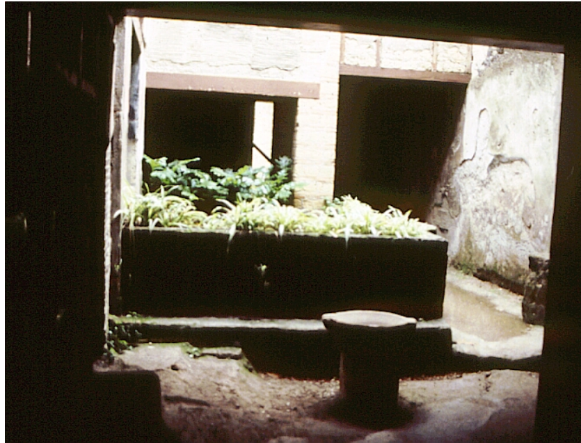
Fig 2 Courtyard and only common space of a crowded multi-resident, multi-storied apartment building, known as the Casa a Graticcio in Herculaneum, first century CE so called because of its use of a common low-standard method of construction using cemented rubble in wood frames. Such apartment houses were notorious for danger of fire and collapse.
