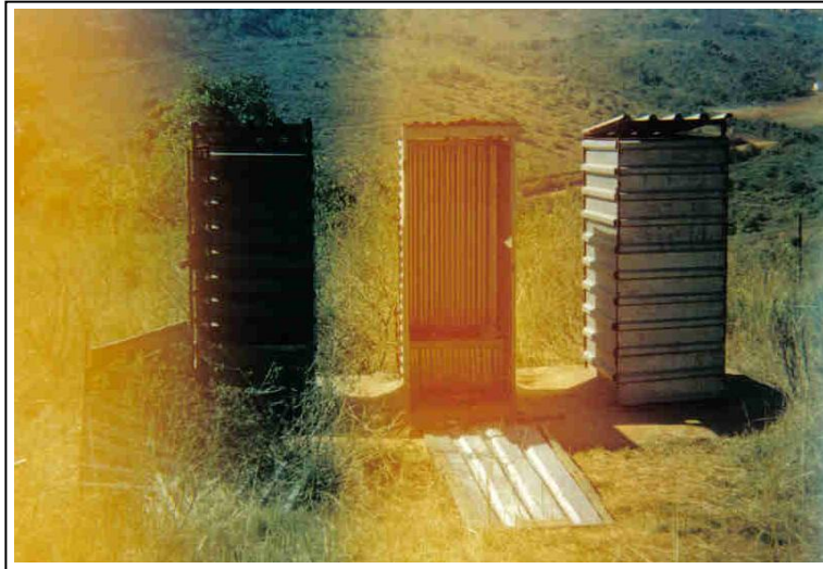
Figure 2.3: Example of pit toilets at a rural public school in Limpopo Province (Netshitahame 1999:82)
