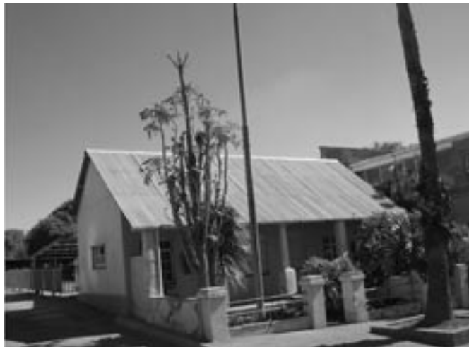
fig.3.23 Existing Building 1: Residential building, currently a security office
