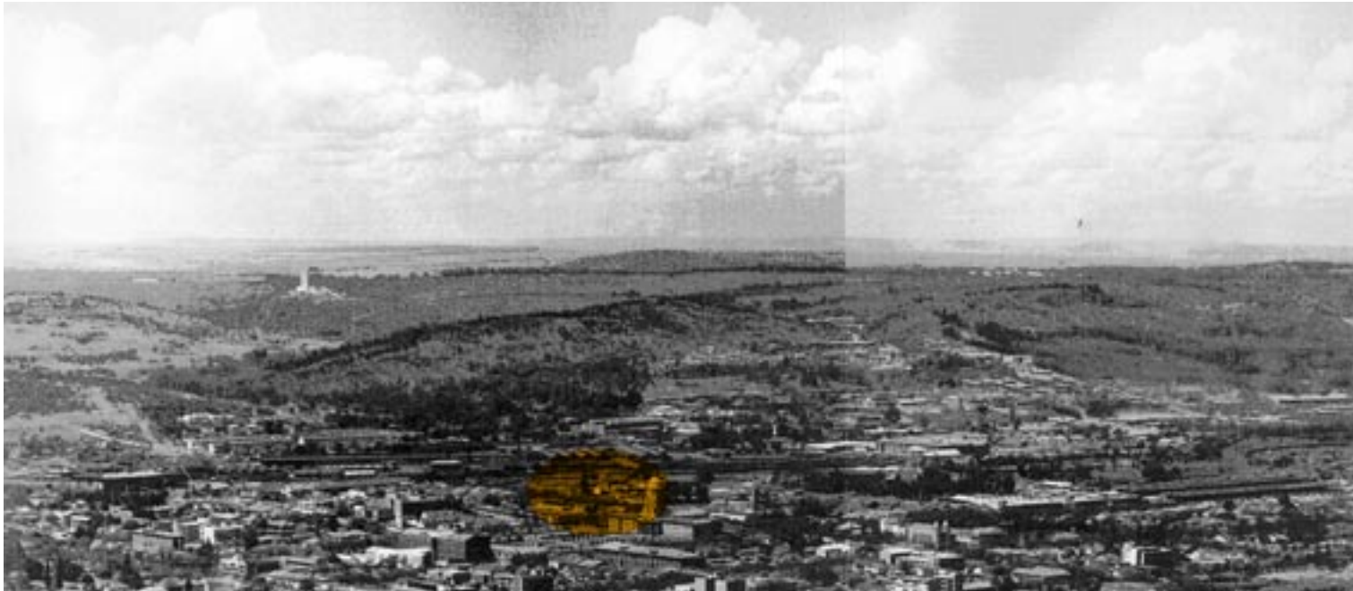
fig.3.20 SANAF Aerial Photograph of Pretoria in early 1900's (exact date
