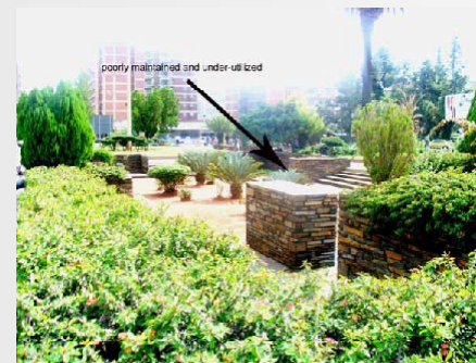
Figure 2.1.1 Poorly maintained sunken garden
