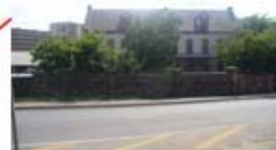
Figure 1.4.13 Old NZASM printing storage, now Intersite offices.
