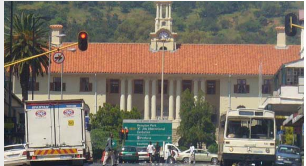
Figure 1.3.5 Pretoria station viewed from Paul Kruger street.
