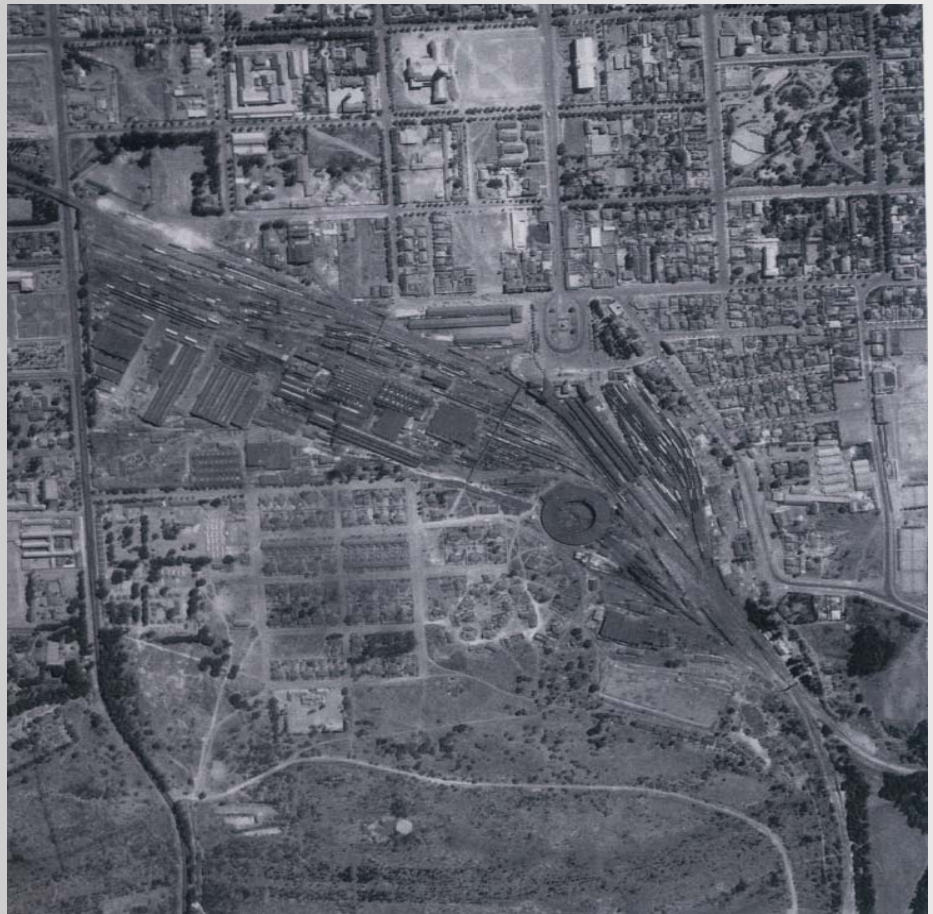
Figure 1.2.7 Salvokop aerial photograph of 1937. (Bakker)
