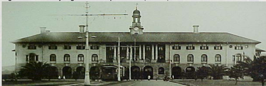
Figure 1.2.4 Sir Herbert Baker designed station building, completed in 1914. (Bakker)
