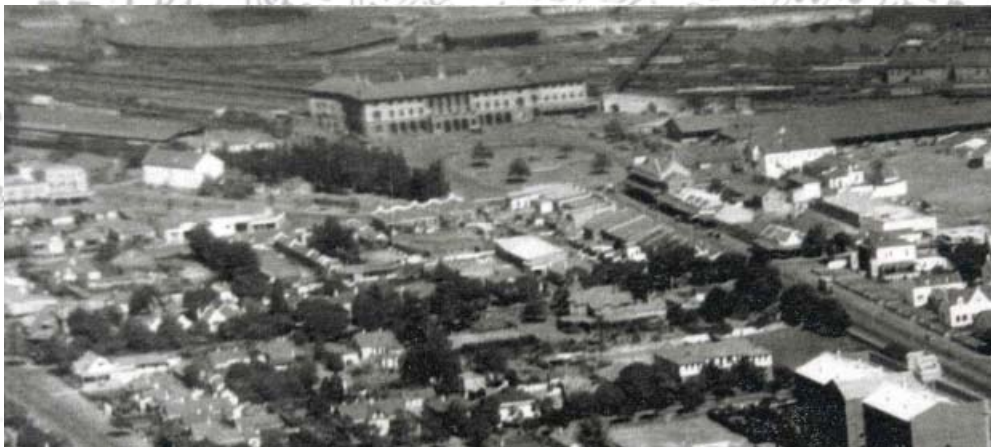
Figure 1.2.1 Pretoria station photo of 1934. (Bakker)
