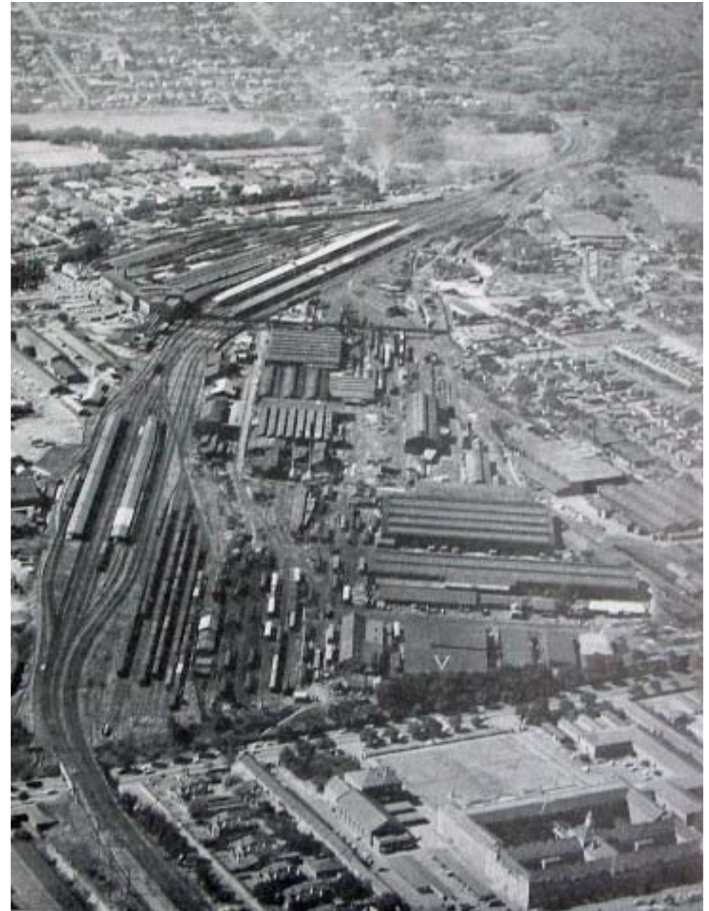
Figure 1.2.2 Aerial view of marshalling yards. (Bakker)
