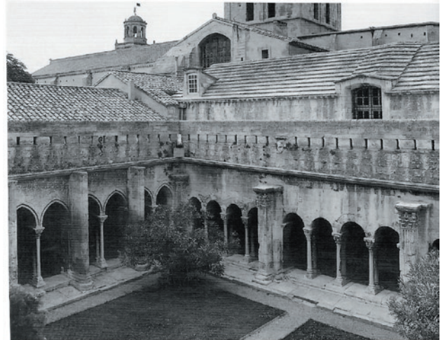
Fig.6_22.Cloister, Abbey of St. Trophine, Fleming, 1995
