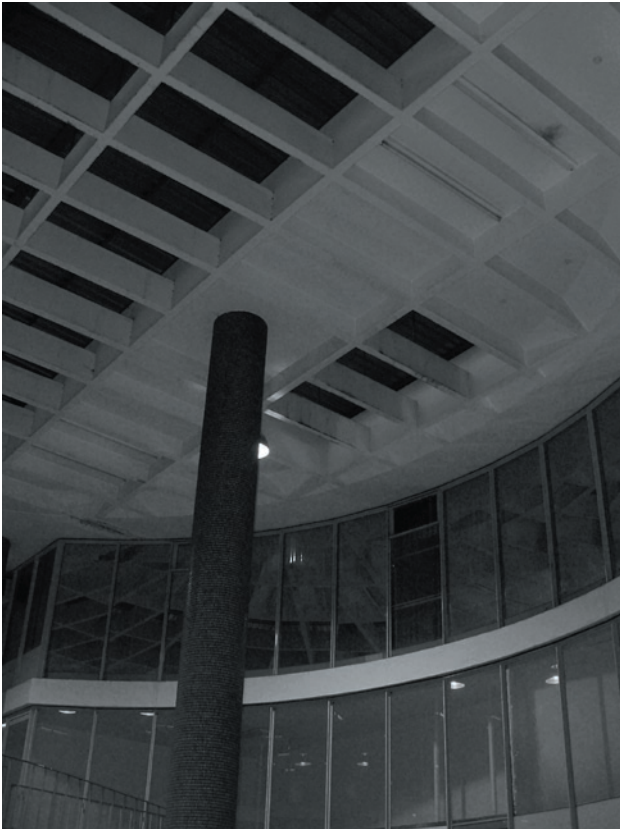
Fig.6_33.Roof over Polleys arcade
