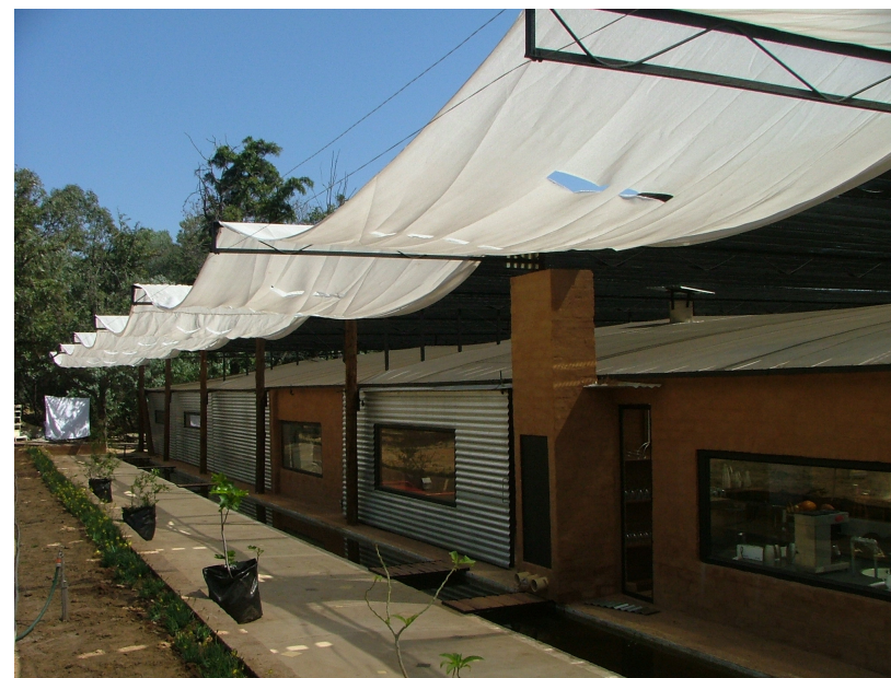
Fig 31: Purple Daisy images: Green house polythene as roof covering, and the combination of various materials to create an interesting facade (Tumubweinee, 2006)
