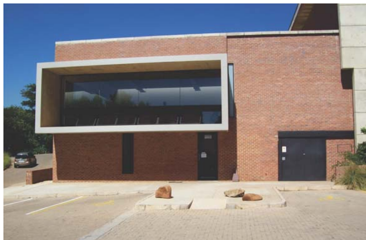
fig. [40] BAY WINDOW ON NORTHERN ELEVATION FACEBRICK AND CONCRETE ENVELOPE
