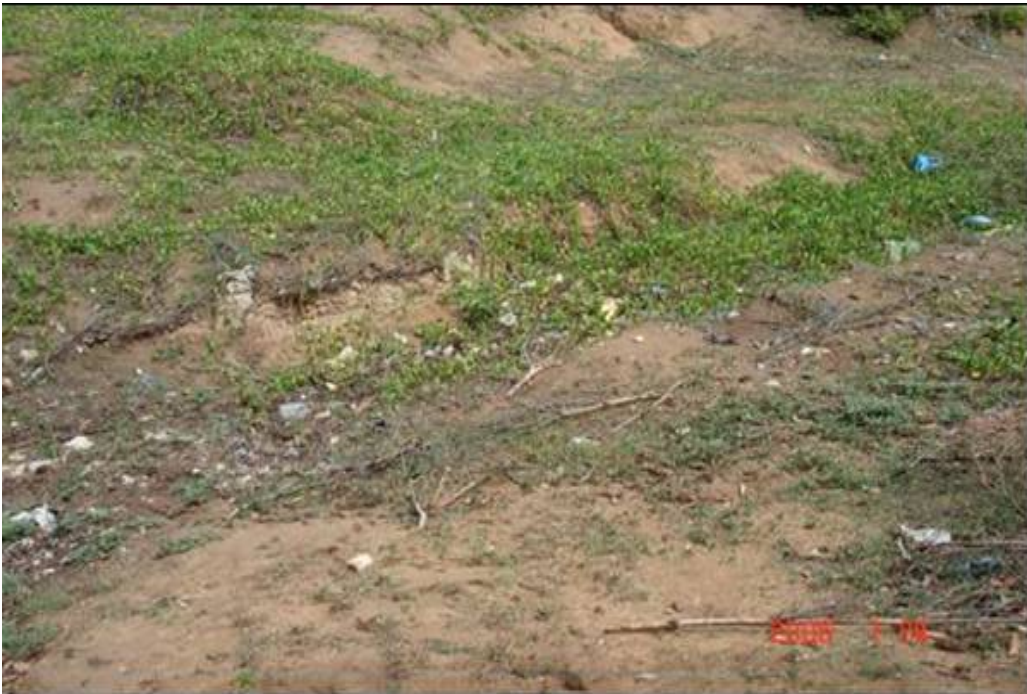
Picture 5: Installation destroyed by some members of the community just weeks after its building in Nacala-Porto district Photo taken by researcher during data collection
