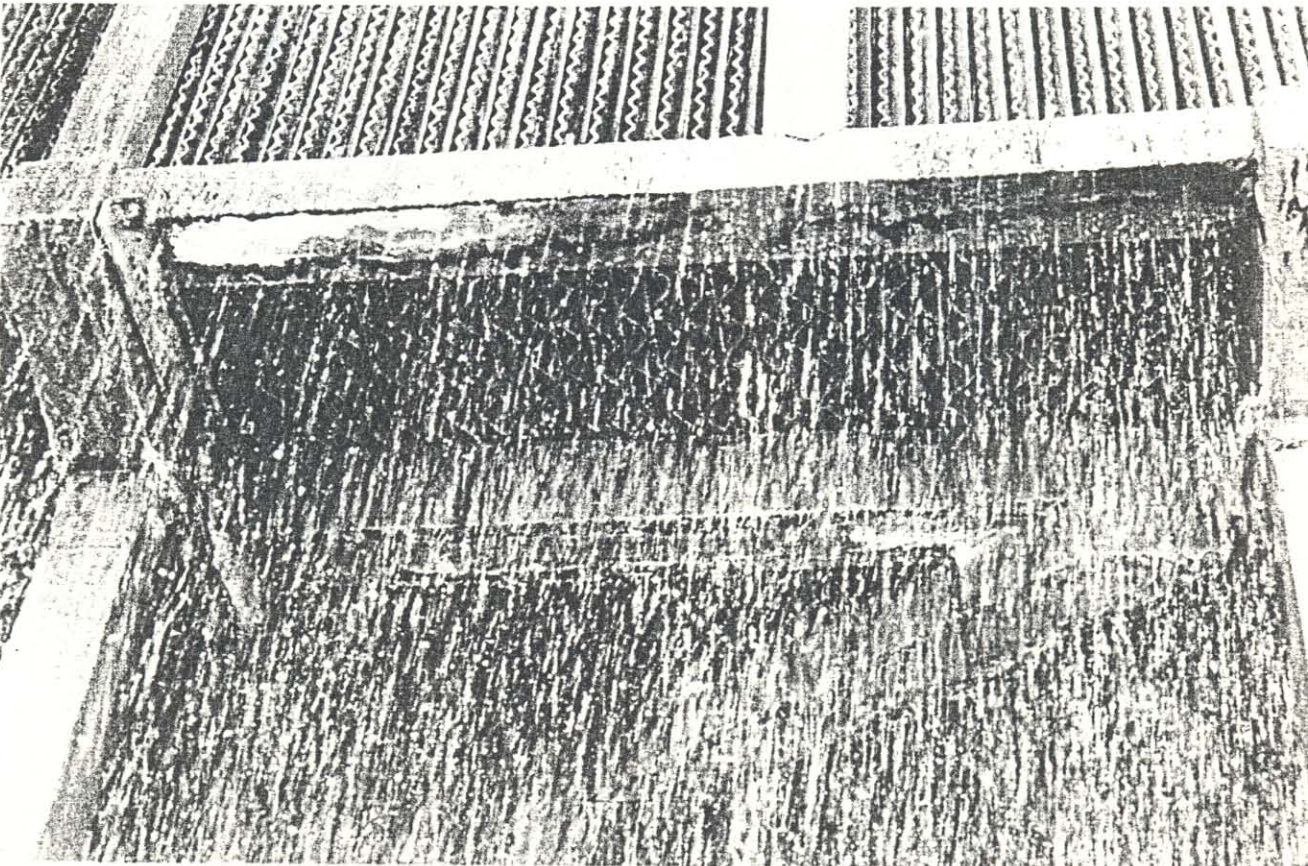
Figure 4.6: Biofouling deposits at Grootvlei Power Station on cooling tower packing before biodispersant/biocide treatment (A) and packing clear of biofouling deposits after three weeks of treatment (B).
