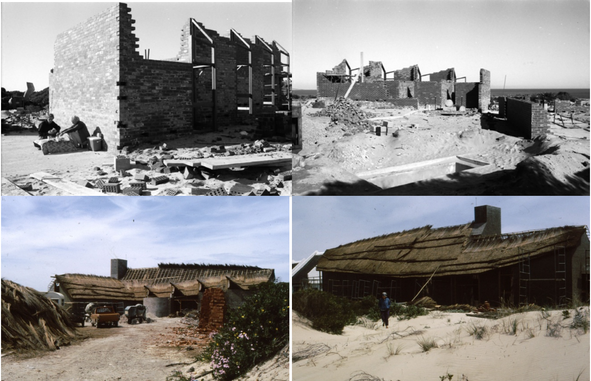
Figure 8.35. Top left: The Fagans picnicking alongside the partly constructed building. Top right: Walls constructed to roof height. Bottom left: Roof under construction viewed from site entry point. Bottom right: Roof under construction as viewed from sea edge (All Fagan archive job no. 8011, slide collection IC).
