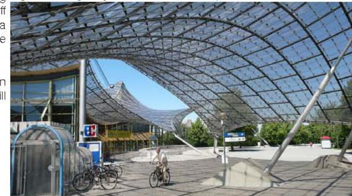
FIG 7.3 Munich olympic stadium roof (Nerdinger 2005:266)
