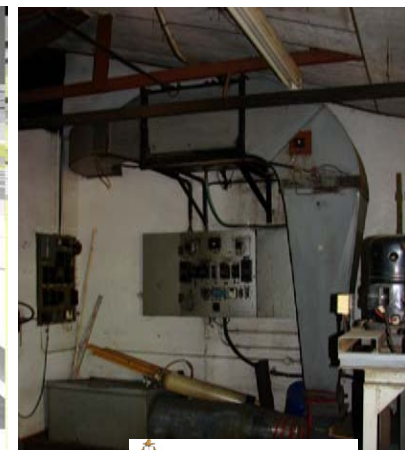
FIG 4.31 Bateman building interior
