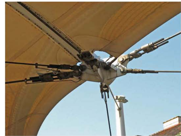
FIG 7.6 Urban-Loritz Platz Straßenbahn by Tillner architects in Vienna, Austria clevis-rod assembly
