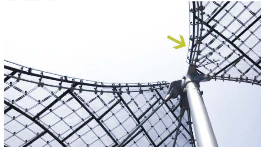
FIG 7.20 Neoprene roof gutter system Munich Olympic stadium, Germany (Nerdinger 2005:268)
