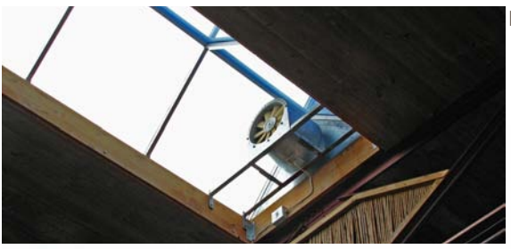
FIG 5.20 Skylights and extractor fans in main hall
