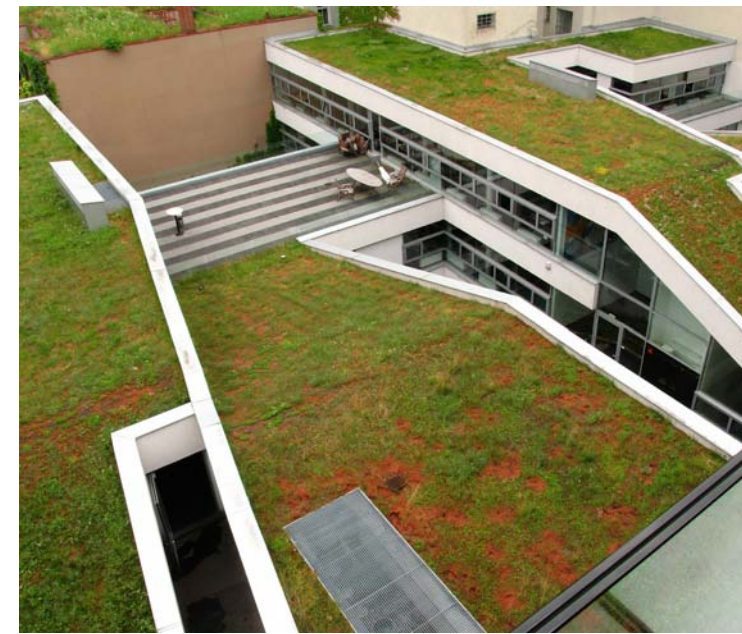
FIG 4.38 Office and residential building at Wimbergergasse, Vienna. Designed by Delugan Meissl associated architects (2001)
