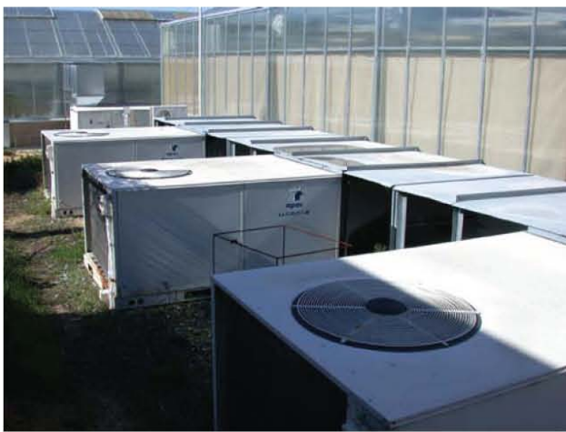
FIG 7.24 Evaporative cooling units and heat exchangers
