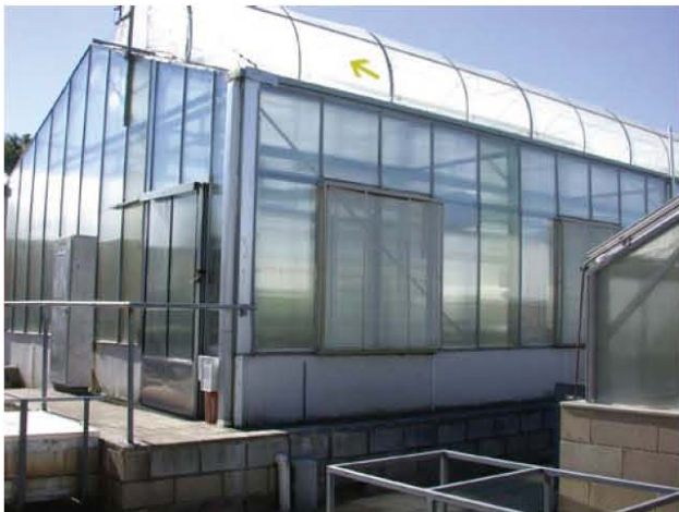
FIG 7.25 Evaporative cooling units cold air release ducts
