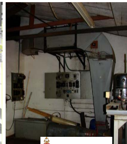
FIG 4.31 Bateman building interior
