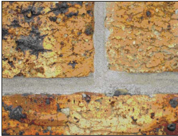
Jointing mortar on the southern facade
