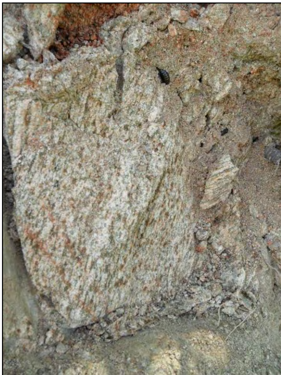
Figure 12: Very soft residual granite
