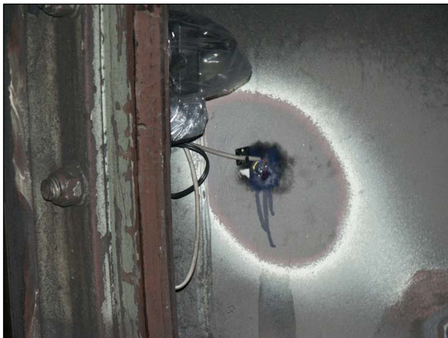
Figure 3.2: Wireless bridge amplifier mounted on the ingo-outgo ring
