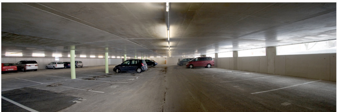
Photo 2.6.1 Flat soffit of a 16m span Cobiax flat-slab, Freistadt, Germany
