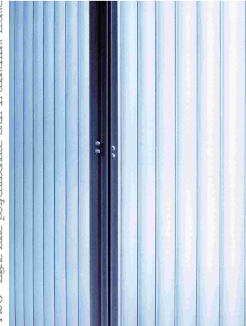
126 Light blue polycarbonate skin in aluminium frame
