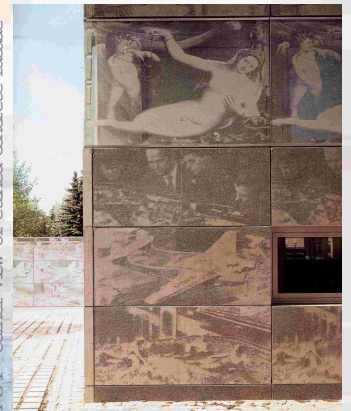
1.31 Corner view of etched concrete facade
