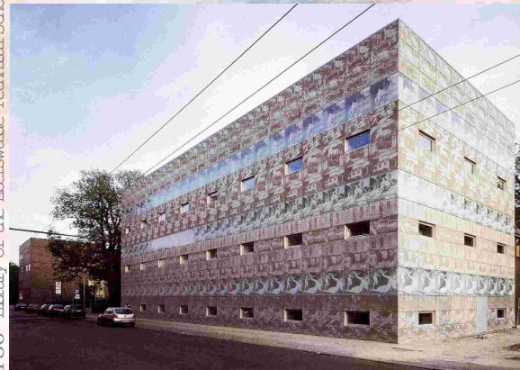
1.31 Corner view of etched concrete facade
