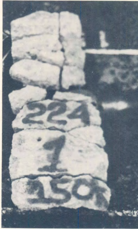
(a) Upper subbase layer cracked and fractured after 17 255 repetitions with 150 kN single wheel load.
