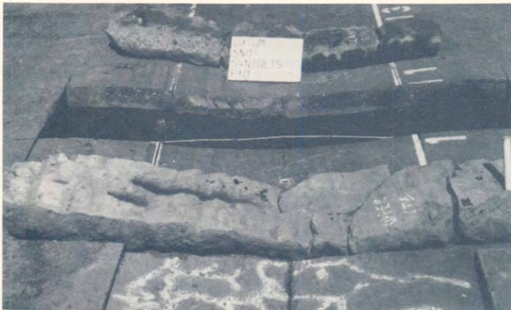
(b) Recovered upper subbase material from Section 2. Note the thinner subbase inside the trafficked area.
