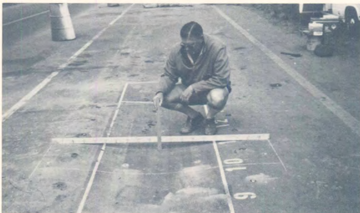
(c) Surface condition of Section 2 after Excess Pore Water Pressure (EPWP) state.
