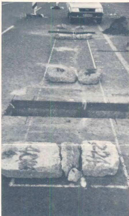
(c) General view of recovered subbase layers on SECTION 2.
