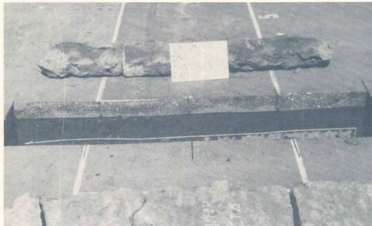
(b) Cross profile on Section 2 after the dry state. No deformation recorded on road surface.
