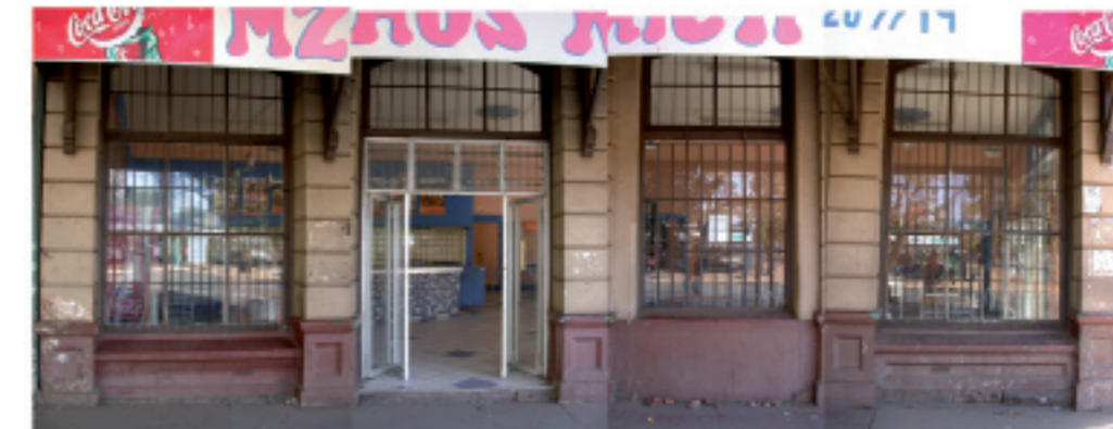
Figure 2.20: Corner Building ground floor facade in 2007
