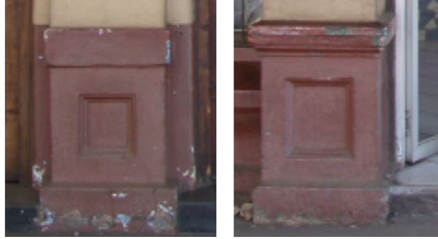
Figure 2.16: South Building column base (left). Figure 2.17: Corner Building column base (right).
