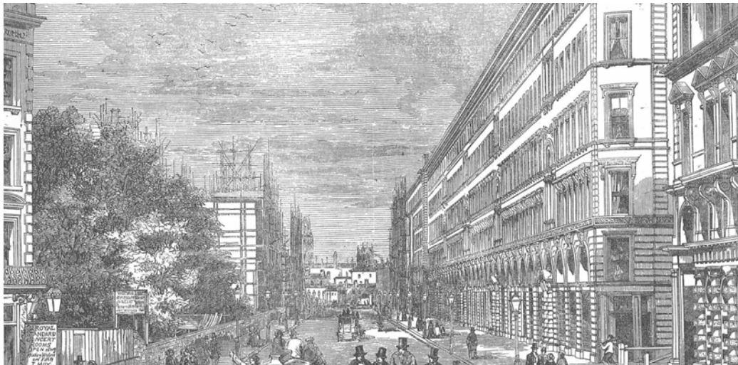
Figure 5.5 Apartment houses in Victoria Street, London, by Henry Ashton, 1852-54. General view looking east
