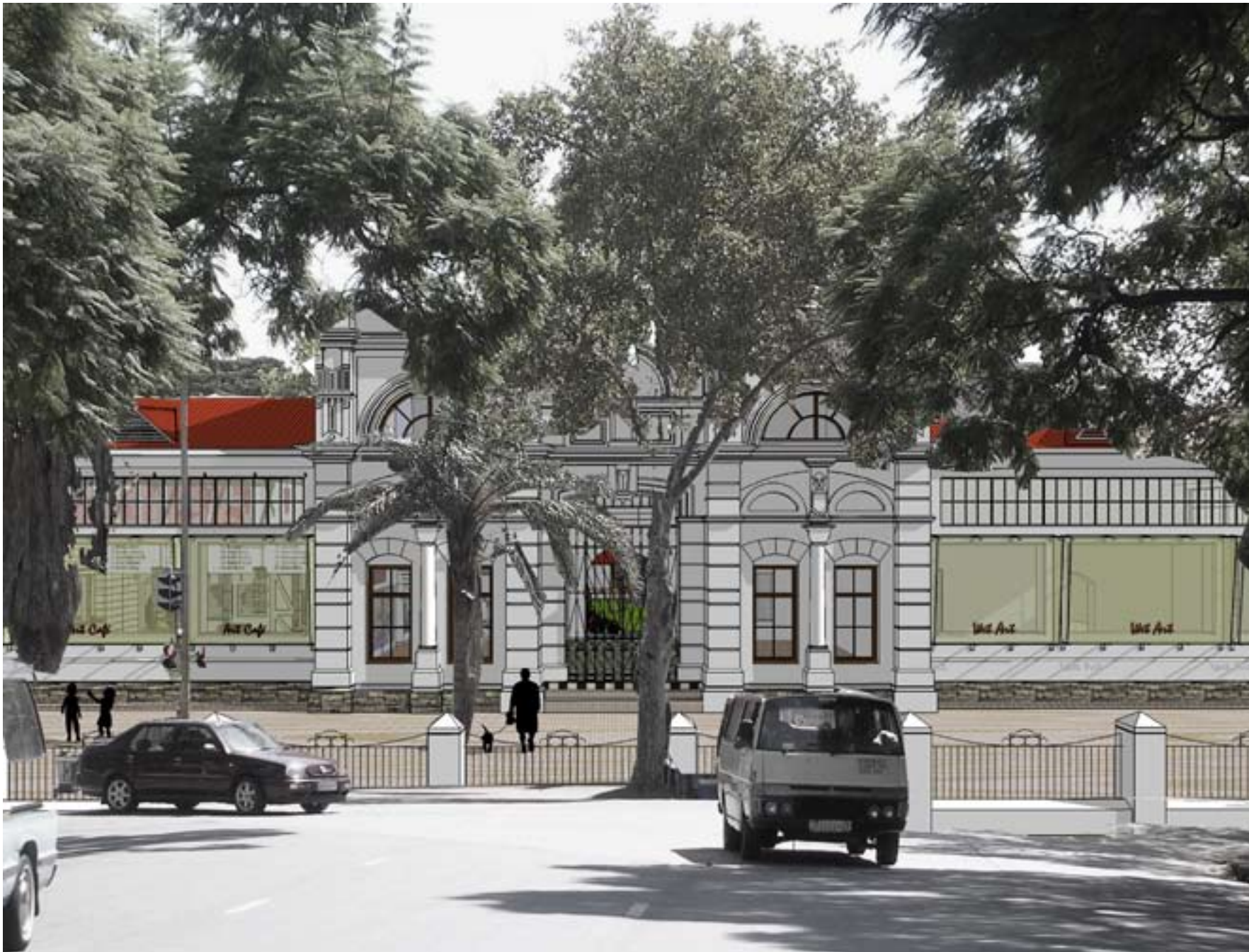
Figure 90(e): Enhanced communication between the exterior and interior
