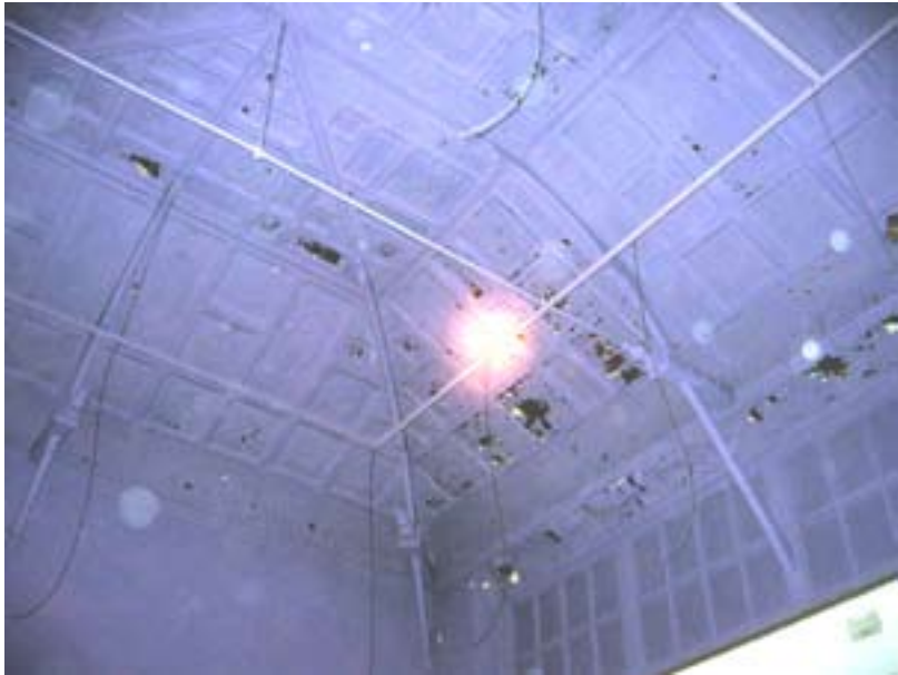
Image 18: The only vaulted pressed steel ceiling in the building, painted purple
