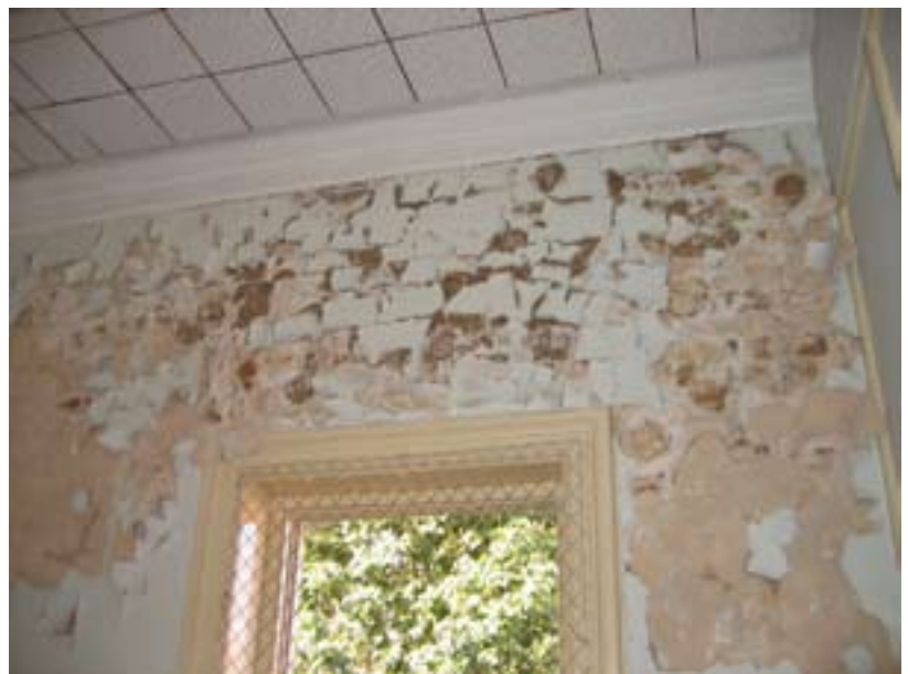
Image 17: The PVA paint layer is peeling off the lime-based paint. (This photo was taken in the northern upper wing, but also applies to the 'tower' first floor.)
