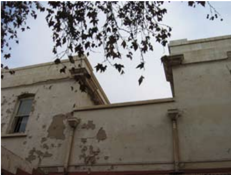
Image 28: One standard sash window is placed on each floor in the 'towers'
