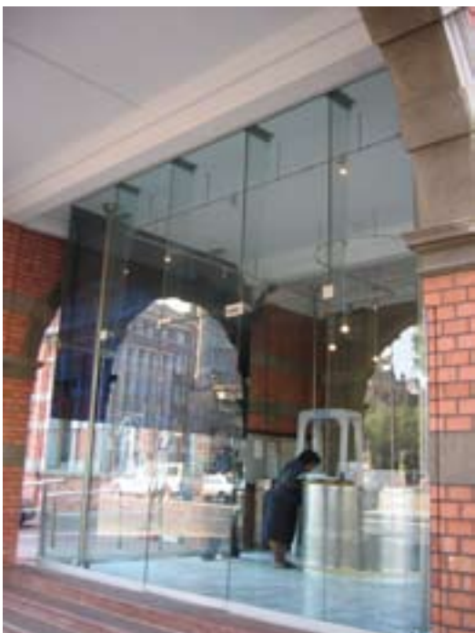
Figure 59: Close-up view of glass partition
