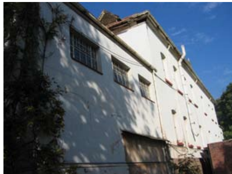
Image 29: Three later added steel windows can be found on either end of the northern wing
