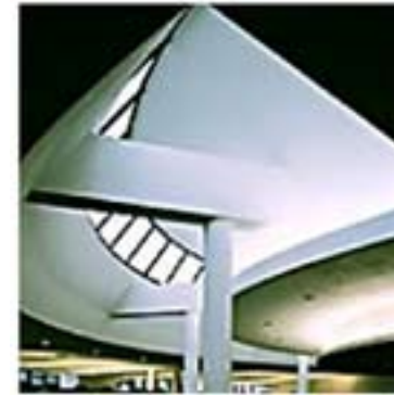
Figure 35: Green painted ceiling to prevent glare
