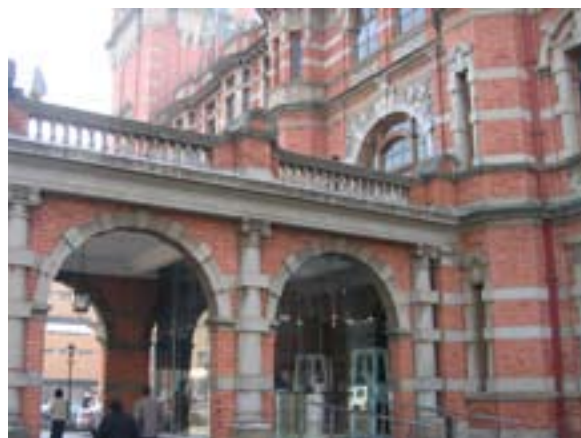
Figure 60: Portal seen in wider context
