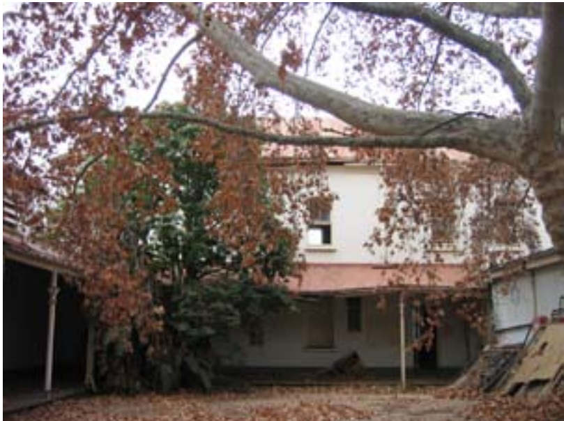
Image 4: The courtyard addition (right wing in photo) ruins the courtyard space
