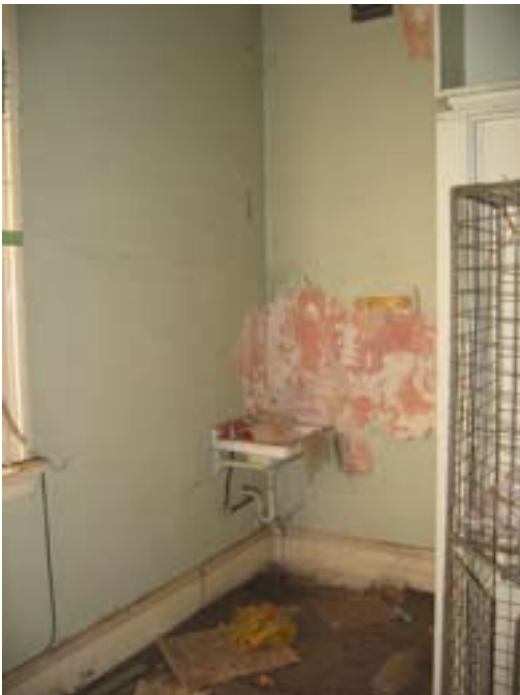
Image 44: A hand basin is found in the eastern 'tower'
