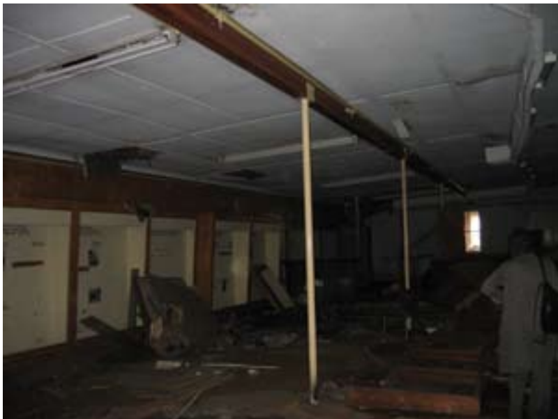
Image 48: The interior courtyard addition is left damaged by water and lack of maintenance
