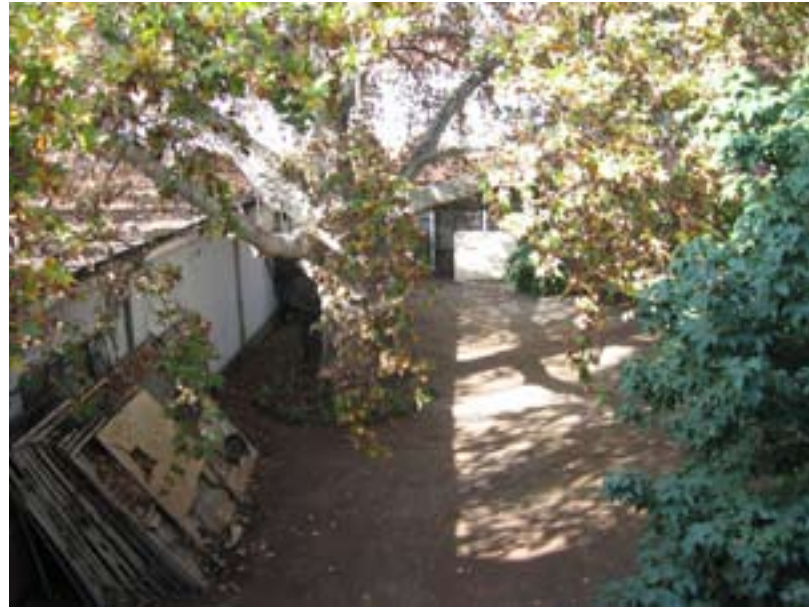
Image 4: The courtyard addition (left wing in photo) ruins the courtyard symmetry and atmosphere
