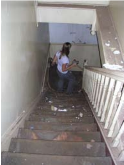
Image 14: Staircase leading up to the 'tower' first floor
