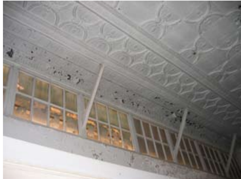
Image 19: The most expensive pressed steel ceiling found in the east wing
