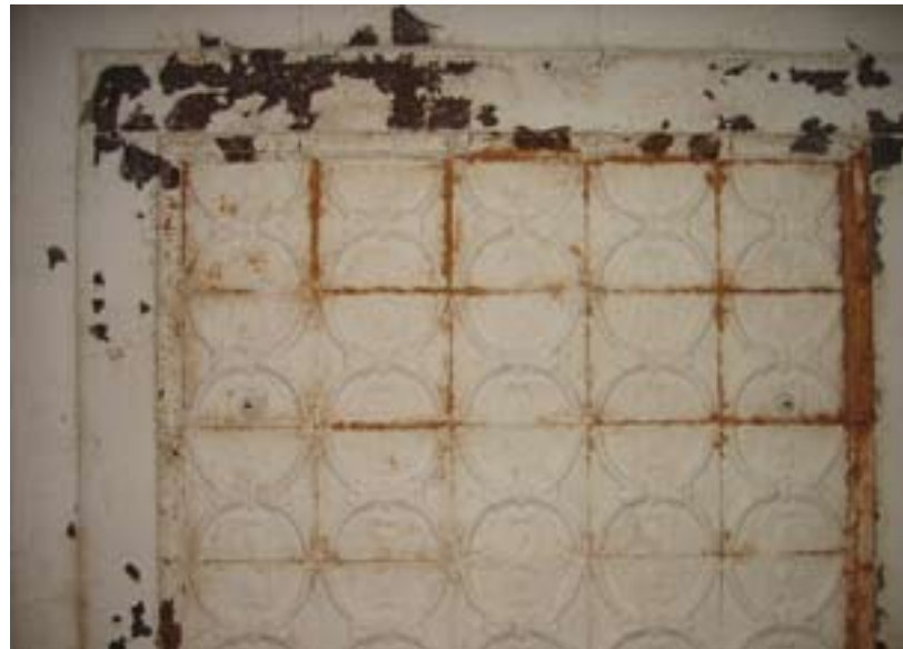
Image 21: The pressed steel ceiling in the foyer
