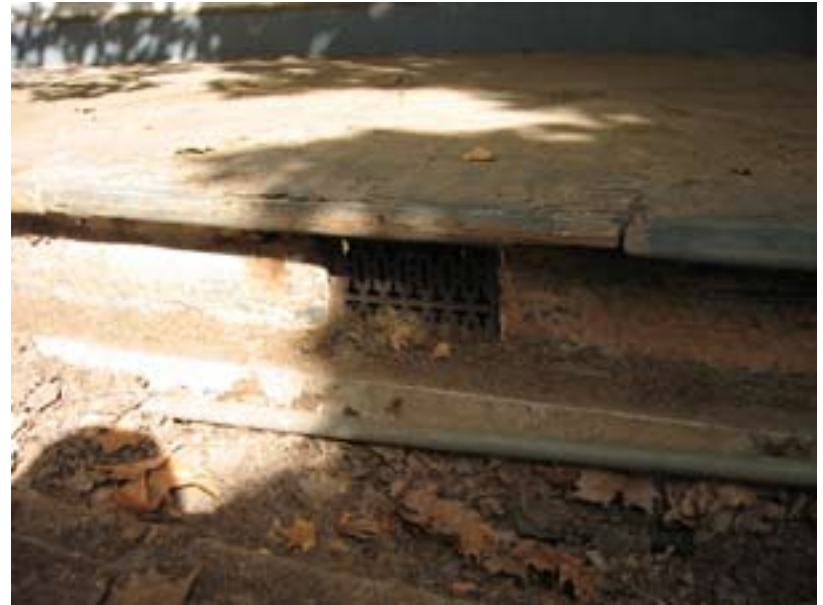
Image 15: Cast iron air vents are found all along the building exterior
