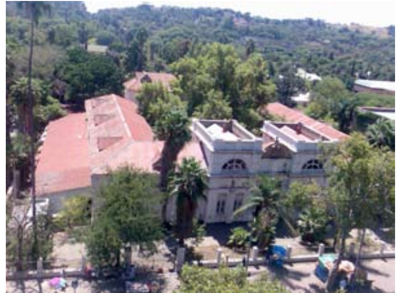
Image 47: A chimney can be seen on either 'tower' roof
