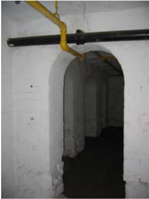
Image 46: Sewage and other pipes run through the basement
