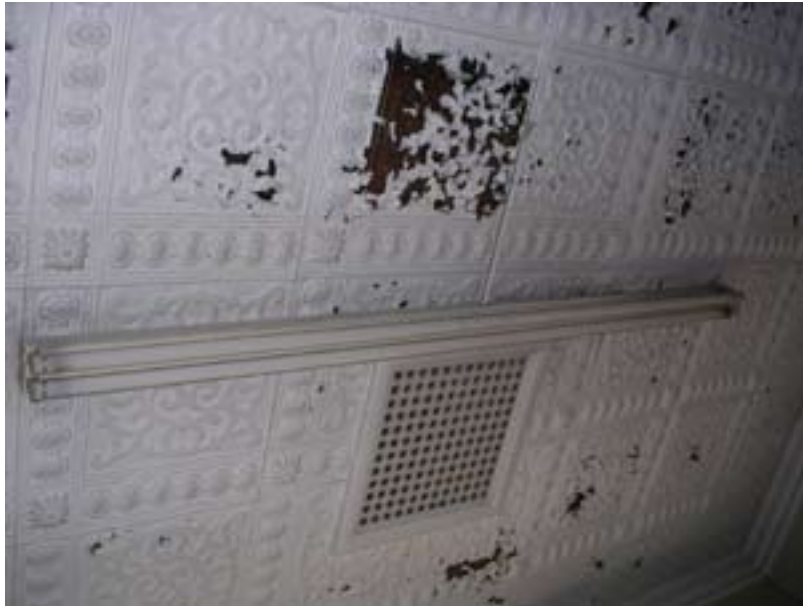
Image 22: Pressed steel ceiling in the 'tower' first floor
