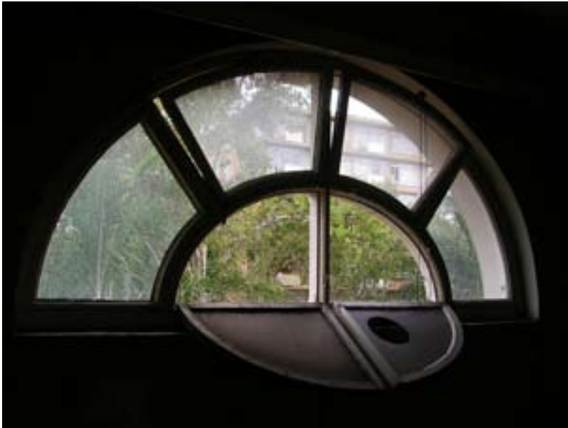
Image 30: A half round window is placed on every first floor of the front facade 'towers'
