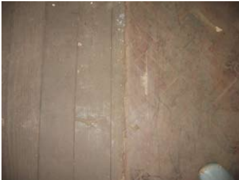
Image 24: The original 'Oregon Pine' timber floor was later covered with a layer of parquet flooring
