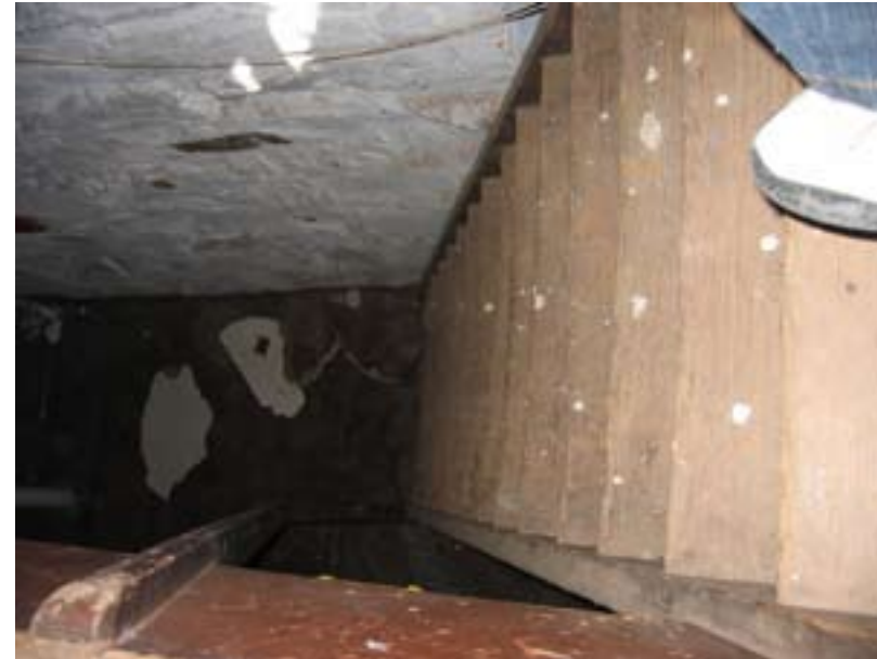
Image 13: A steep staircase leads down into the basement
