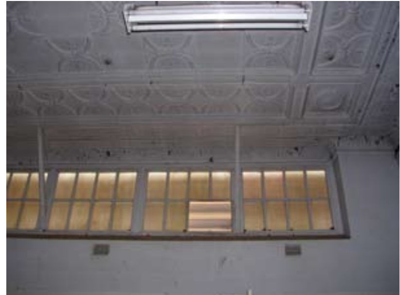
Image 31: Clerestory windows line many facades of the building
