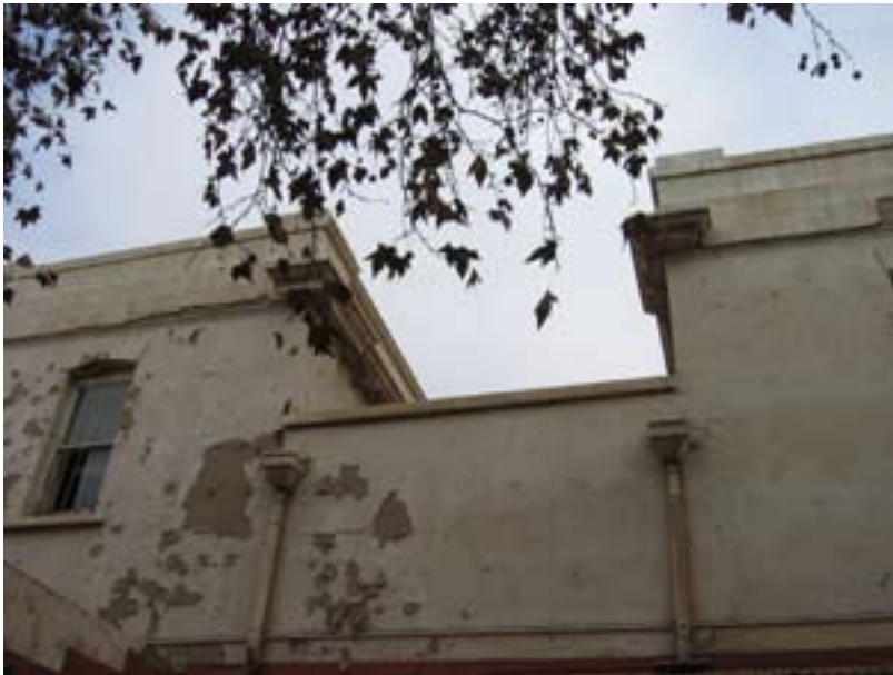
Image 28: One standard sash window is placed on each floor in the 'towers'
