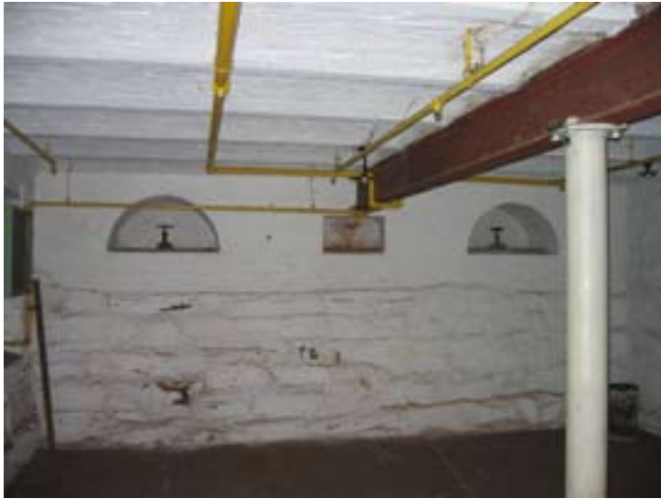
Image 10: Open area in basement
