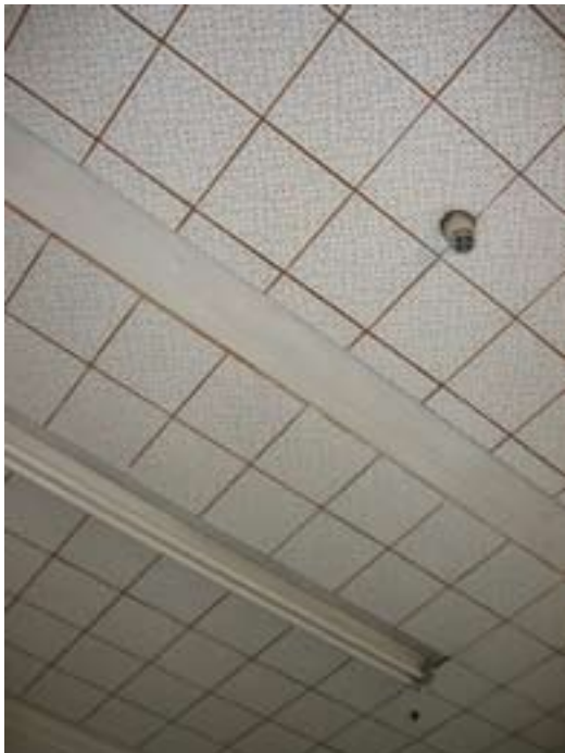
Image 20: The original 'Baltic Deal' timber ceiling is concealed by the later added acoustic panels
