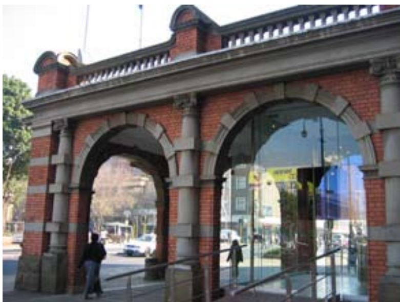
Figure 58: Side view onto glass-enclosed portal
