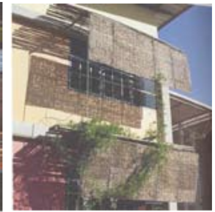
Figure 54: Locally manufactured sun shaders
