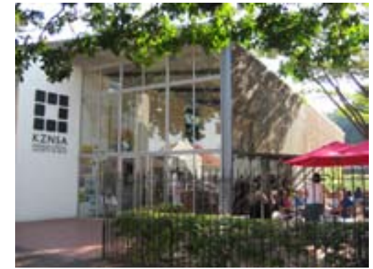
Figure 61: Street view onto gallery
