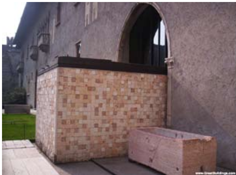
Figure 39: Detail of walls revealing different time layers through different use of materials
