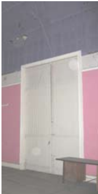
Figure 19: 'Wagon' timber door
