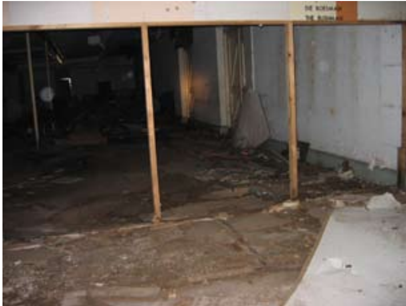
Figure 18: View into courtyard addition
