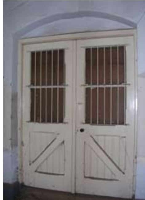
Figure 20: Existing door into courtyard
