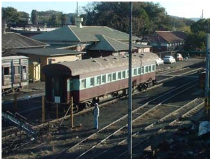
Fig. 7.1 Rails placed directly on to compacted soil. Capital Park, Pretoria
