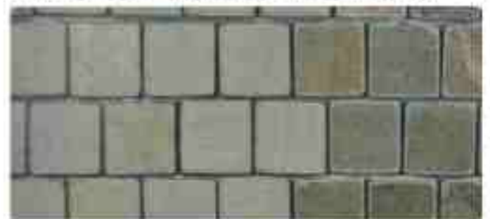
Fig.156 Floor Finish (Architecture SA 2007:3)
