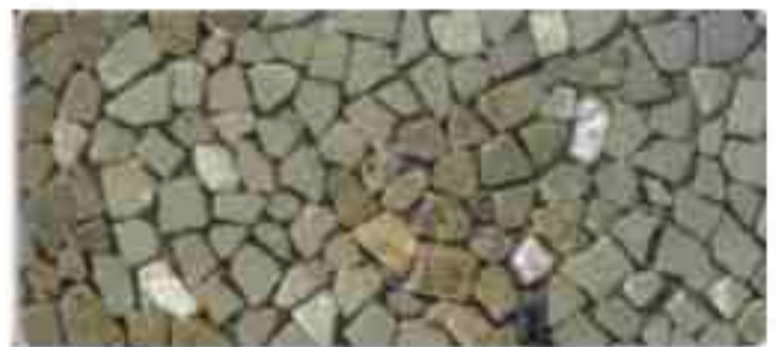
Fig.155 Floor Finish (Architecture SA 2007:3)
