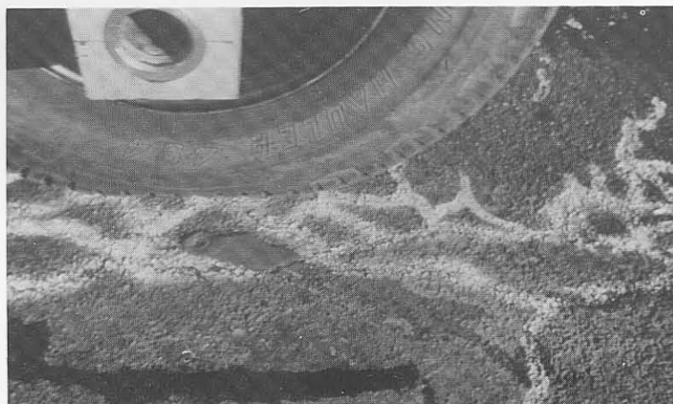
(c) Pumping of the crushed cemented base material.
