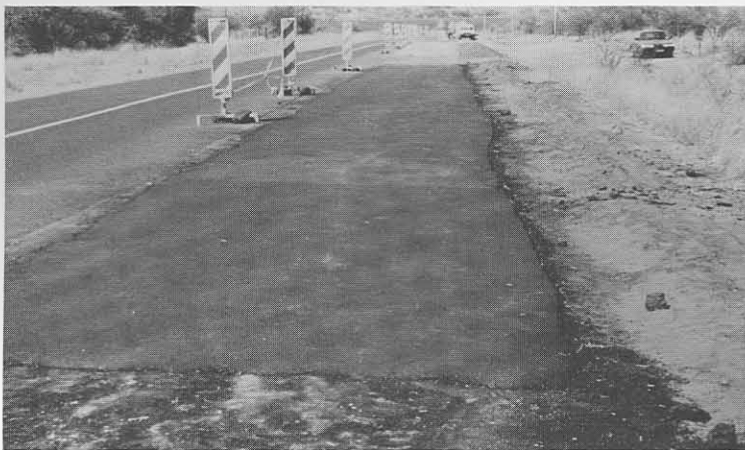
(c) Final surface of the 35 mm asphalt premix section (40 m in length).
