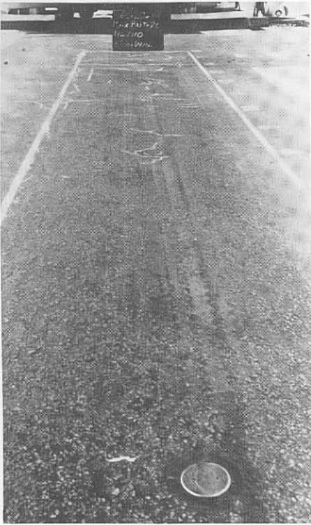
(a) Condition before testing; some fine cracking evident from measuring points 9 to 15 at the start of the test.
