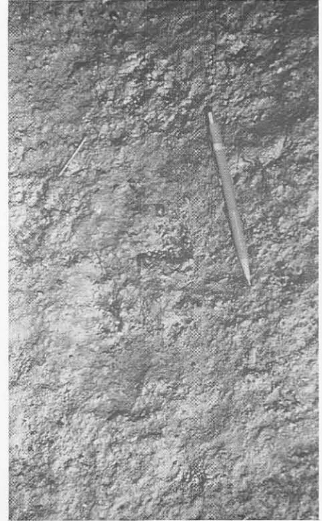
(b) Surface of the precracked cemented base after application of the prime coat.
