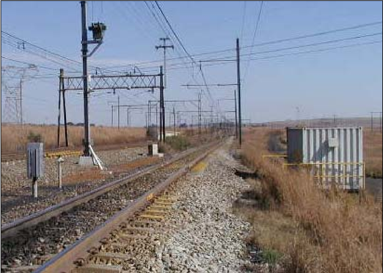
Figure 4-8: A complete unmanned weigh-in-motion weighbridge.
