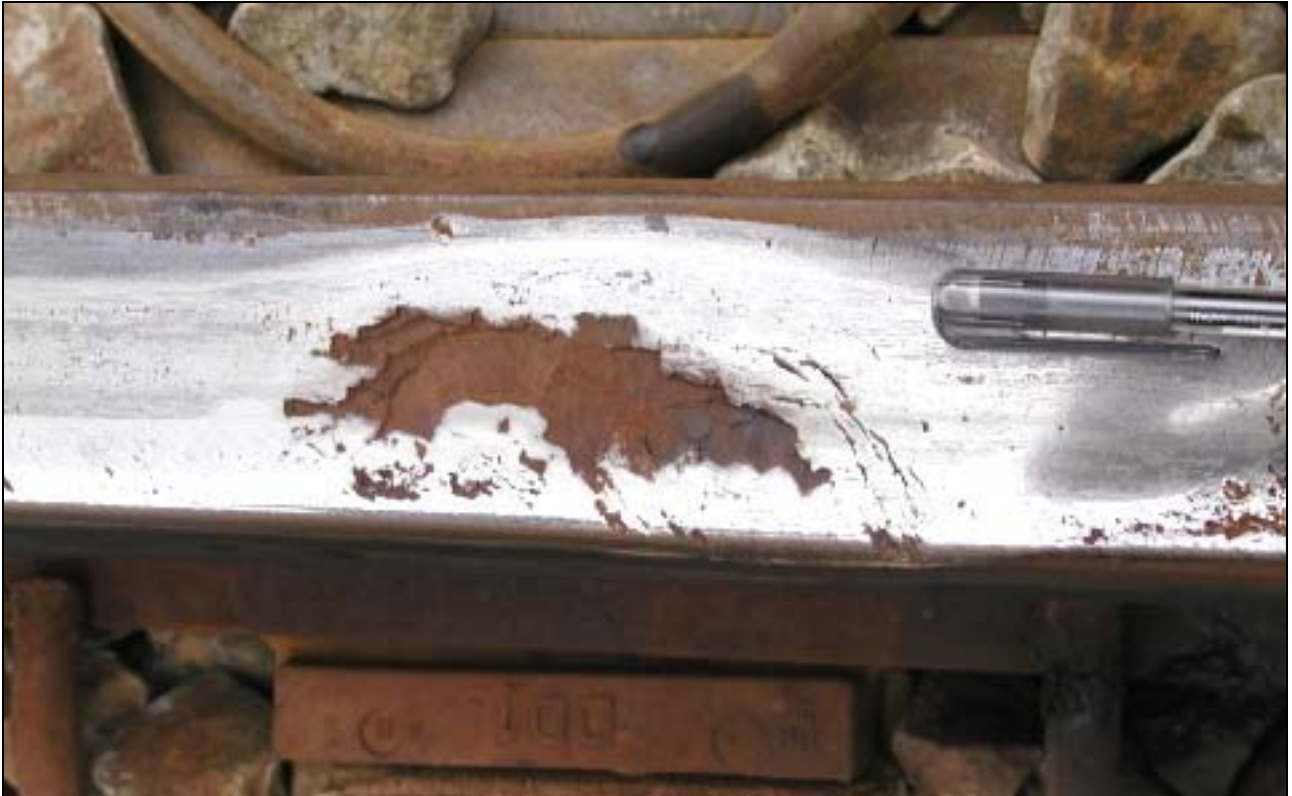
Figure 4-1: Skid mark on rail running surface
