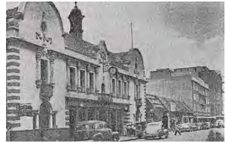
Figure 4: Photograph of the old Town Hall with the City Centre building unbuilt (Pretoria News, 19 March 1954).
