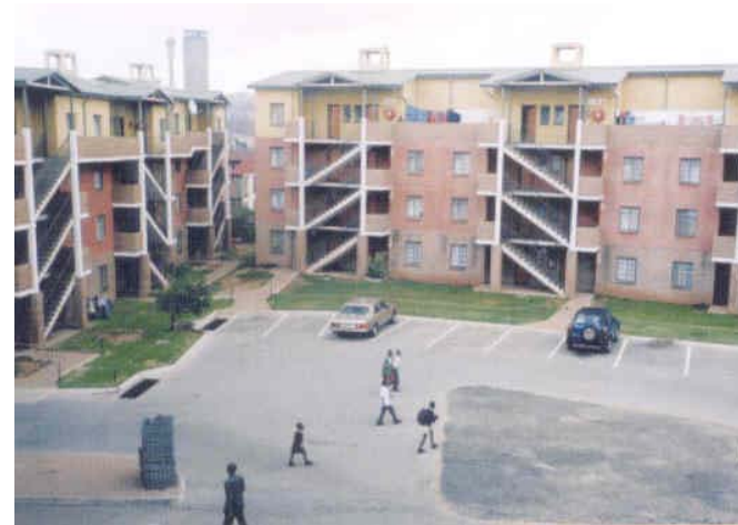
Figure 4.2.2.1 The blocks overlooking the courtyard (The Social Housing Foundation, Issue 3, 2005:4)
