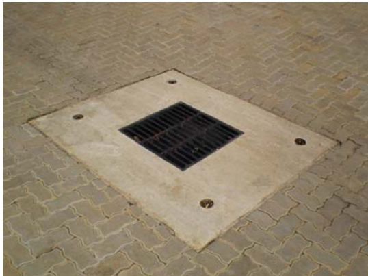
Figure 6.7.8.1 Stormwater drain
