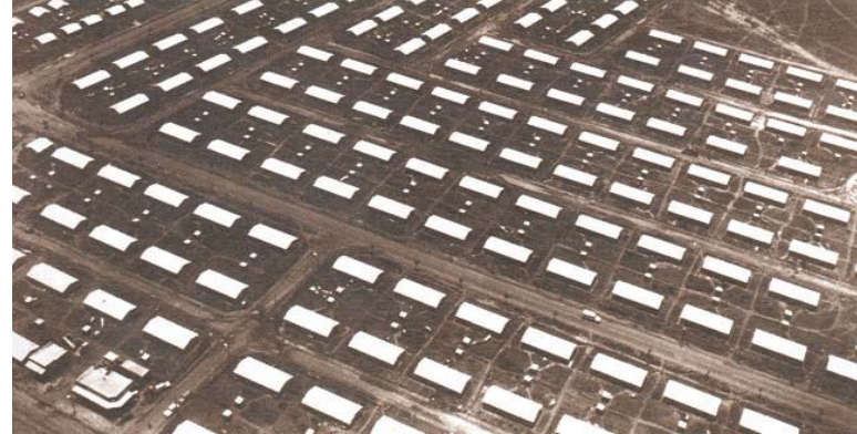
Figure 1.0.1 Standards housing for disadvantaged communities designed by Apartheid regime.
