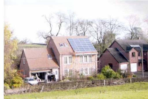
Figure 6.3.2.1 Photovoltaic panels on to of the roof tiles (Toggweiler, 1993, 51)
