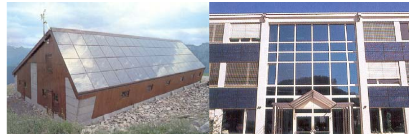
Figure 6.3.2.2 Photovoltaic panels as a building element (Toggweiler, 1993, 65-60)
