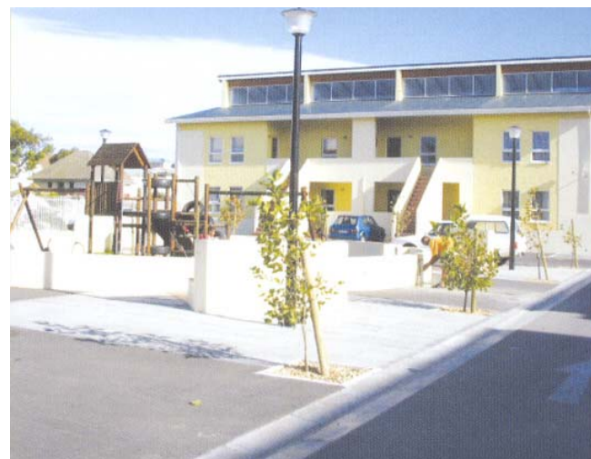
Figure 4.2.1.2 Units overlooking the public spaces (The Social Housing Foundation, Issue 2, 2005:5)
