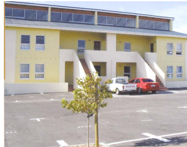
Figure 4.2.1.1 Access to housing units
