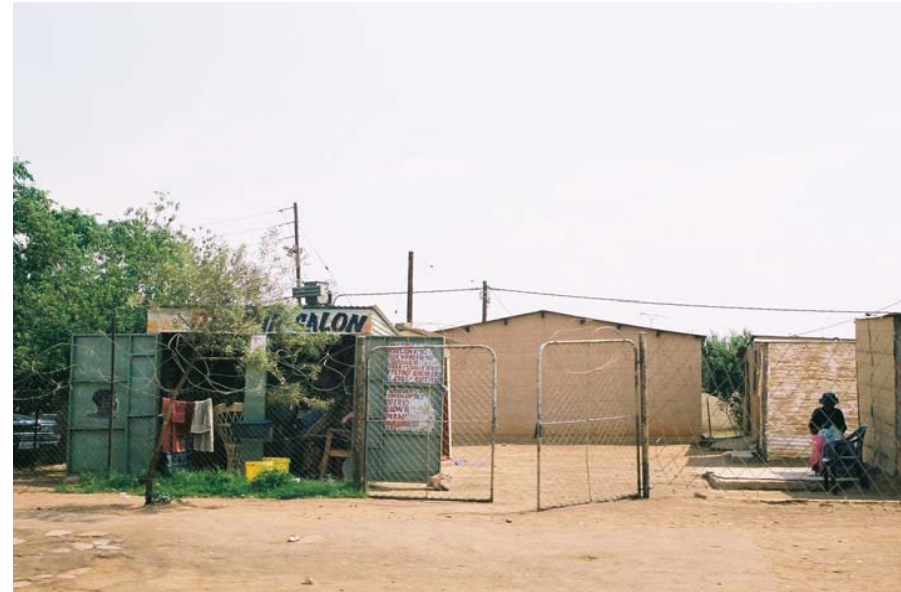
Figure 3.1.1.1 RDP housing with commercial facility (Hair Salon)
