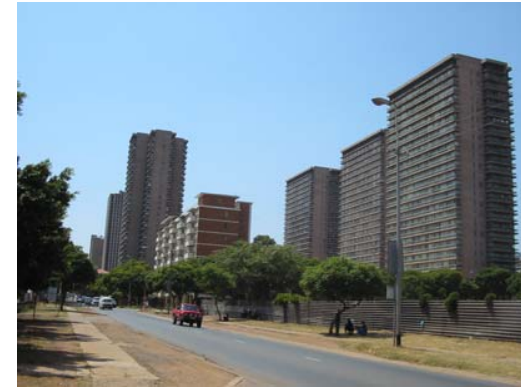
Figure 3.2.2.4 Residential buildings on South side of the site
