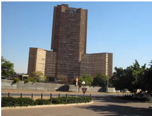
Figure 3.2.2.5 Residential building on South-west of the site
