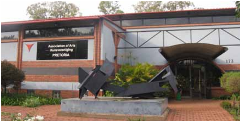
Fig. 1.8.1 Pretoria Arts Association current facility.
