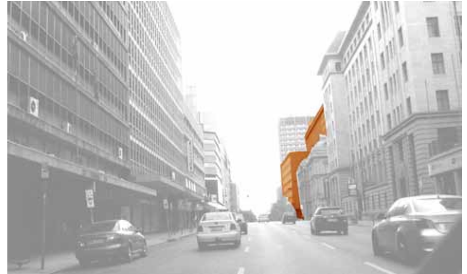
Fig. 3.3.2.2.4 Southern block of the TPA building, facing Pretorius Street.
