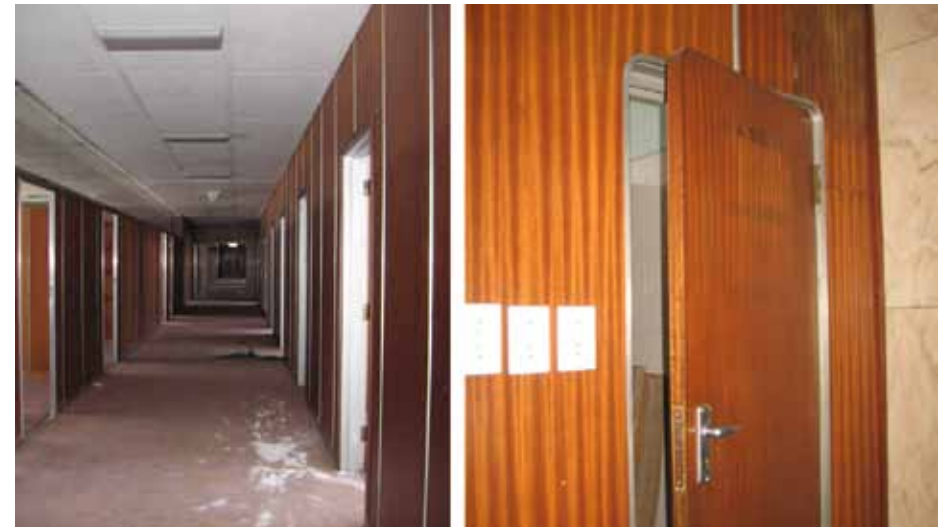
Fig.3.3.2.6.1 Interior partition walls within the TPA building.
