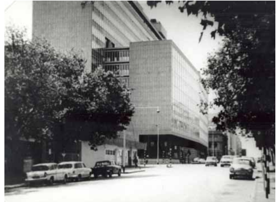
Fig.3.2.1.2 Transvaal Provincial Administration building 1966. [Image: Van der Waal Collection]
