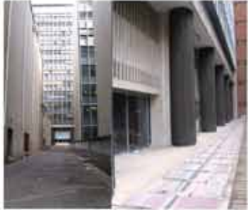
Entrance_ Church Street
