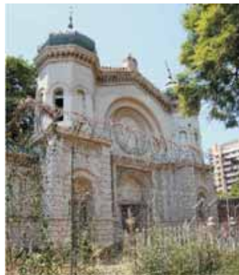
1_34.11 L : The Old Synagogue : Currently it is unoccupied and in a state of disrepair. The Department of Public Works is looking for an appropriate re-use for it.
