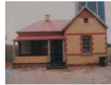
1_34.13 N: Old house : A single storey house with its characteristically corrugated pitched roof, gable wall and stoep. It is currently under renovation and will be serving as offices for the National Library.
