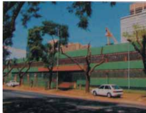
1_34.12 M: SITA Building: A 2 storey building clad with IBR sheeting to its front facade. It houses the government IT department and has its own printing press area.
