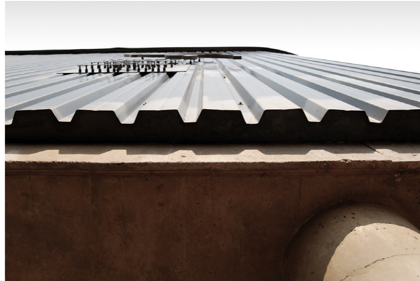
Figure 5.29: Steel sheeting forming shadow line above concrete
