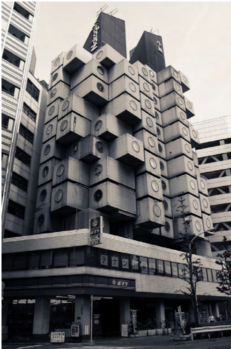
Figure 11.5: Nakagin Capsule Tower , designed by Kisho Kurokawa, 1972. An example of a combination of mechanical flexibility and modular flexibility.
