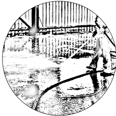
Figure 7.1: Floor being sprayed
