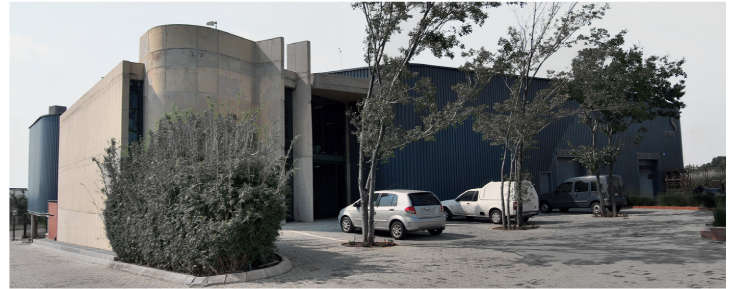
Figure 5.25: View looking southeast showing public entrance of the building
