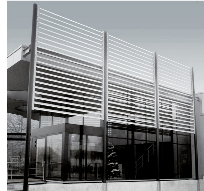
Figure 7.18.3: Photo showing the application of aluminium louvred facade
