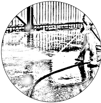
Figure 7.1: Floor being sprayed
