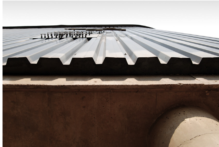
Figure 5.29: Steel sheeting forming shadow line above concrete
