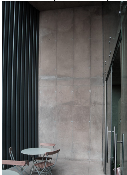
Figure 5.27: Steel sheeting adjacent to concrete wall with shadow gap
