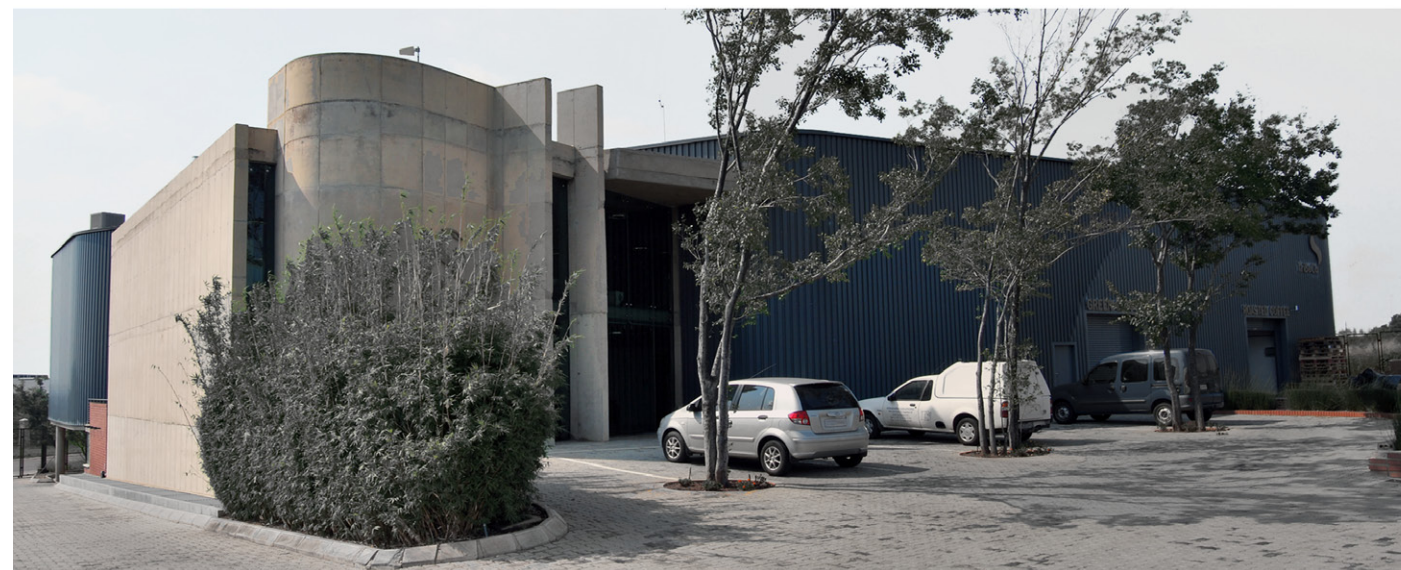
Figure 5.25: View looking southeast showing public entrance of the building
