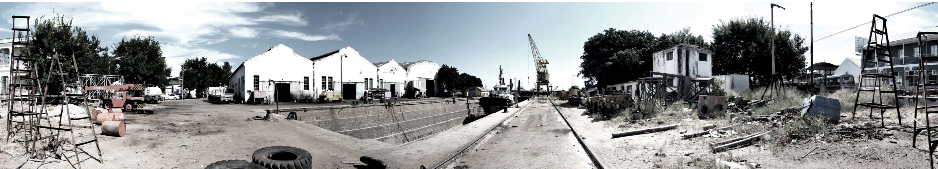
Figure 4.4 (above): Panoramic view of dry dock adjacent to Maputo Fisheries Harbour
