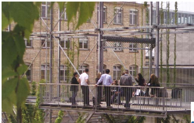
Fig. 67: One of the suspended platforms (Fajardo, 2008: 54).
