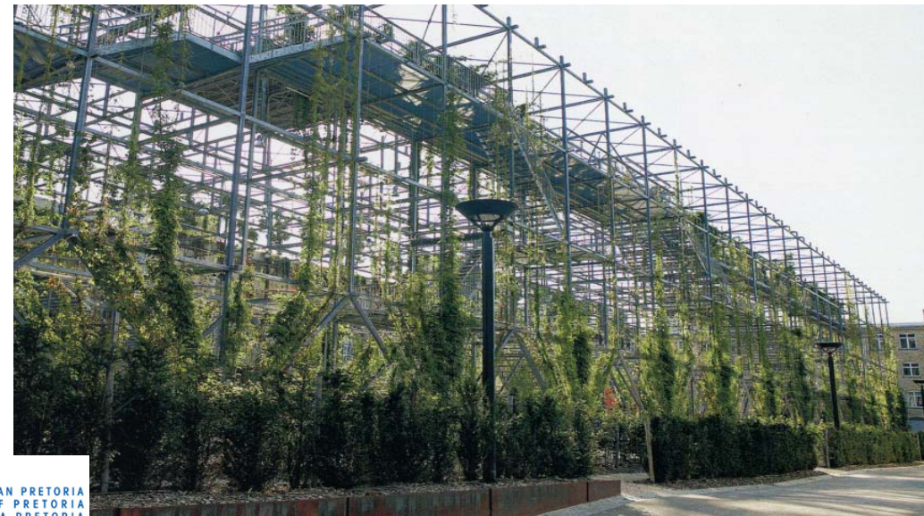
Fig. 68: MFO Park - a steel structure with a cable network for vegetation to envelop the structure (McLeod, 2008).
