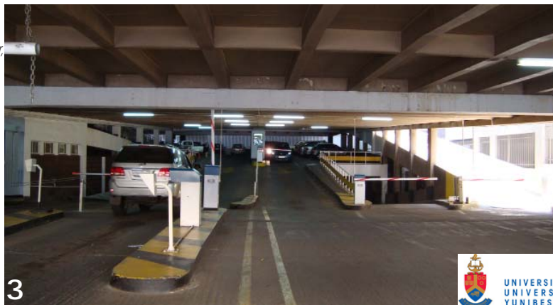
Fig. 33: Municipal arcade with its entrance to the south of the block in Schoeman Street (Author, 2010).
