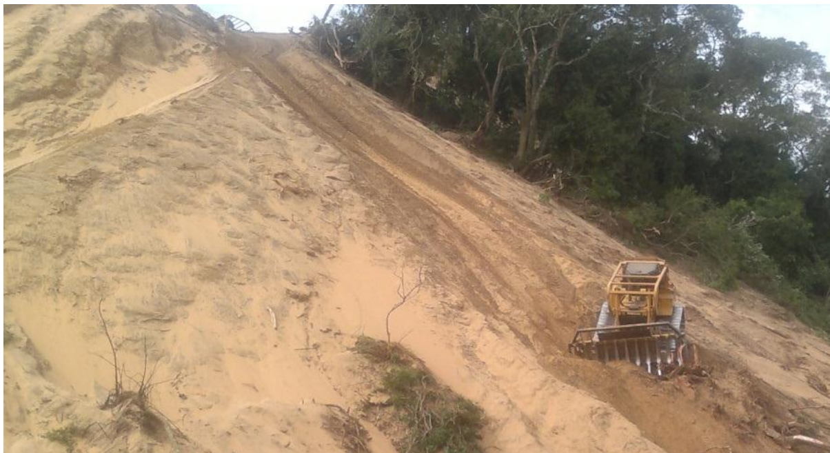
Plate 1. Heavy machinery is used to clear vegetation from the coastal dunes prior to the extraction minerals from the sand.
