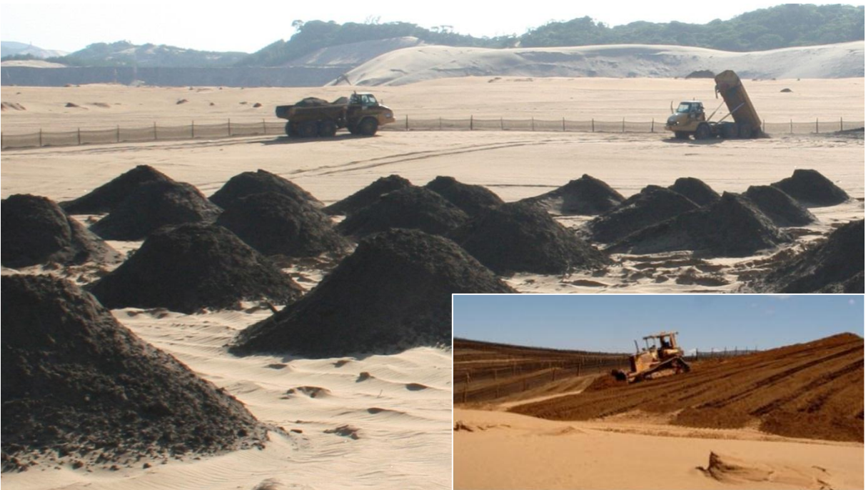
Plate 4. Topsoil collected from cleared areas ahead of the mine is brought and spread over the newly stacked dunes. This is then sown with annuals and indigenous to stabilize the dune as soon as possible with a cover crop. Shade-netting is erected to prevent wind erosion, as well as shade and protect seedlings.
