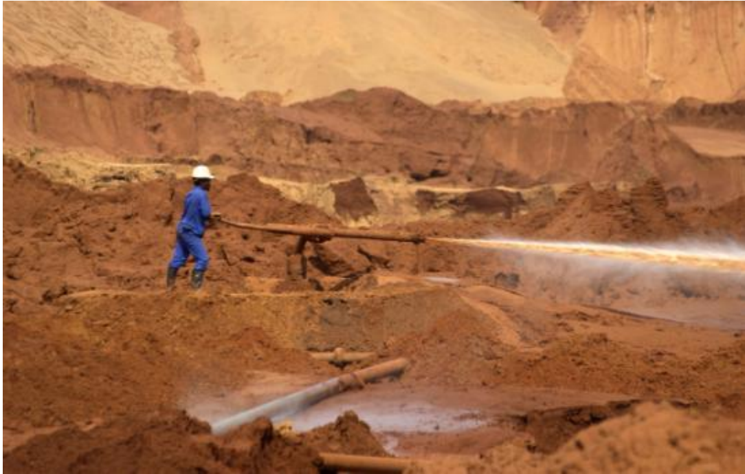
Figure 4. Hydraulic monitor gun at Hillendale mine
