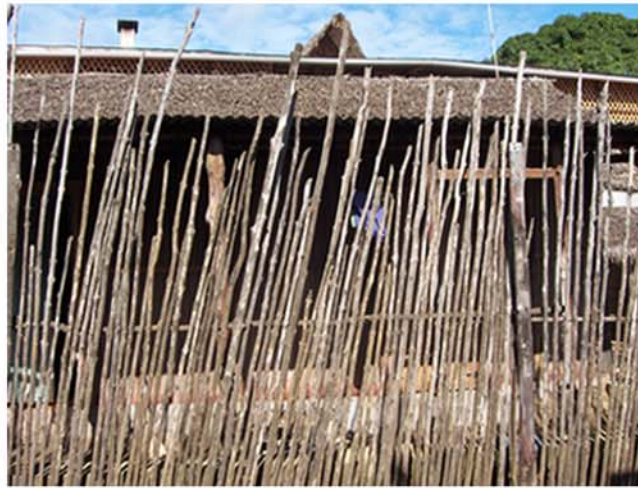
FIG. 171: PERIMETER FENCING MADE OUT OF MANGROVE LOGS (PHOTO: AUTHOR, MARCH 2006).
