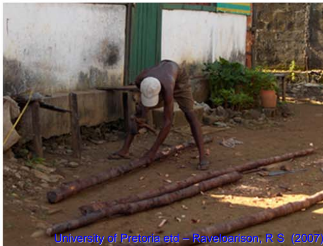
FIG. 172: A FAMILY MAN WORKING ON MANGROVE LOGS TO MAKE A PERIMETER FENCE (PHOTO: AUTHOR, MARCH 2006).
