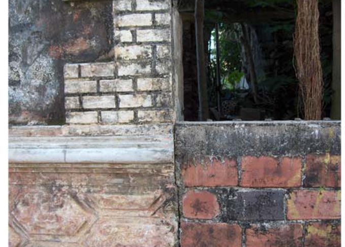
FIG. 174: DETAIL VIEW OF RUINED SODOMA WALL MADE OUT OF FACEBRICKS AND CORAL STONE (PHOTO: AUTHOR, JANUARY 2006).
