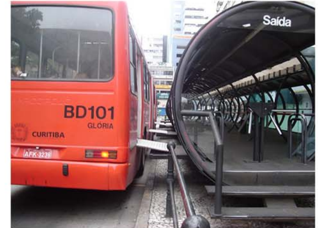
FIG. 82: A CURITIBA BUS STATION (PHOTO: HAJA RASAMBAINARIVO, MARCH 2006).
