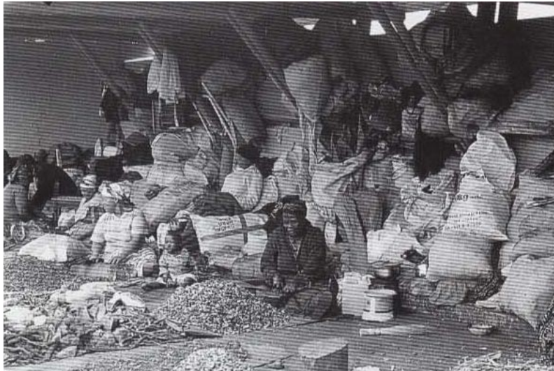
Fig. 3.2 Herb traders under roof structure erected on bridge (Dobson, 2001)
